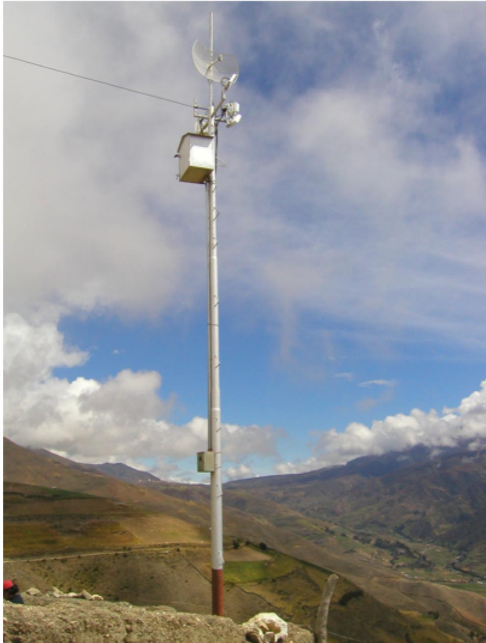
**Often it is less expensive than a tower, and can be built by attaching foot rests to any sizable pipe**
