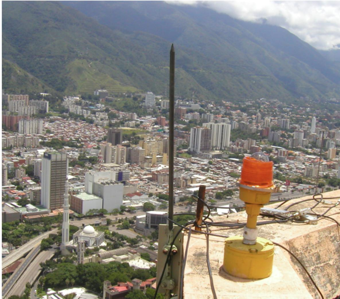
A lightning arrester is a must for any structure elevated above the surrounds. An inexpensive solution is to use a grounding rod properly connected to ground.
