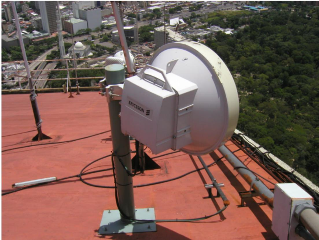
Mounting the antennas close to the edge of the rooftop (on a flat top roof) helps to avoid problems with the latter requirement and with reflections. This should be done at the edge facing the air
