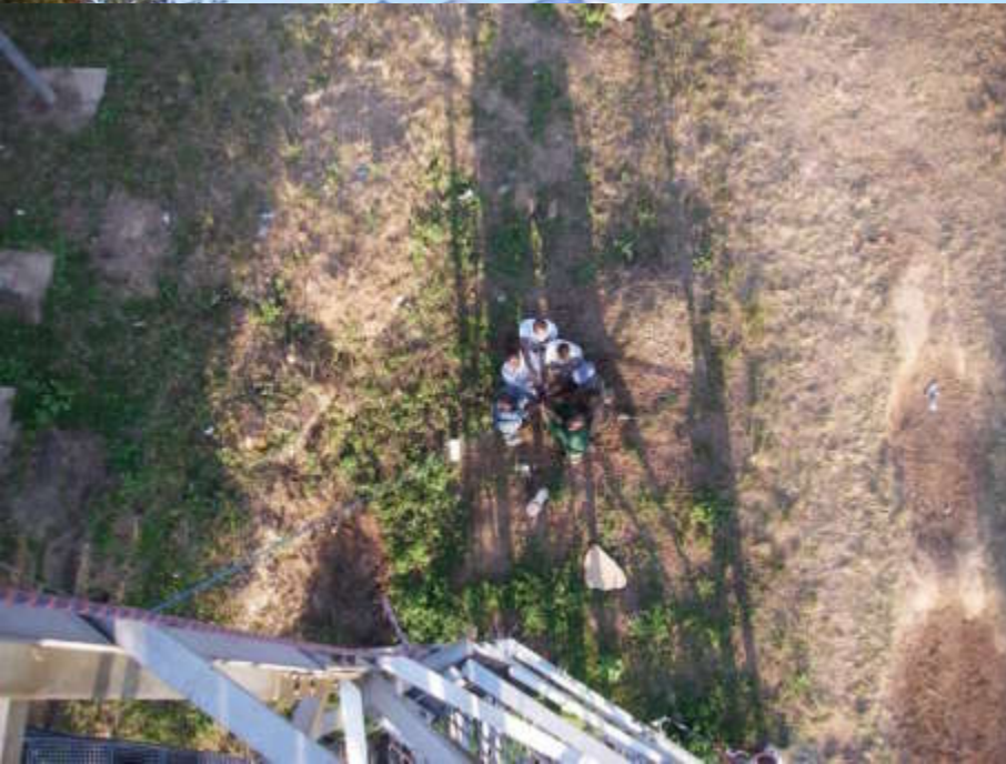
Team work for antenna hoisting in Mangochi
